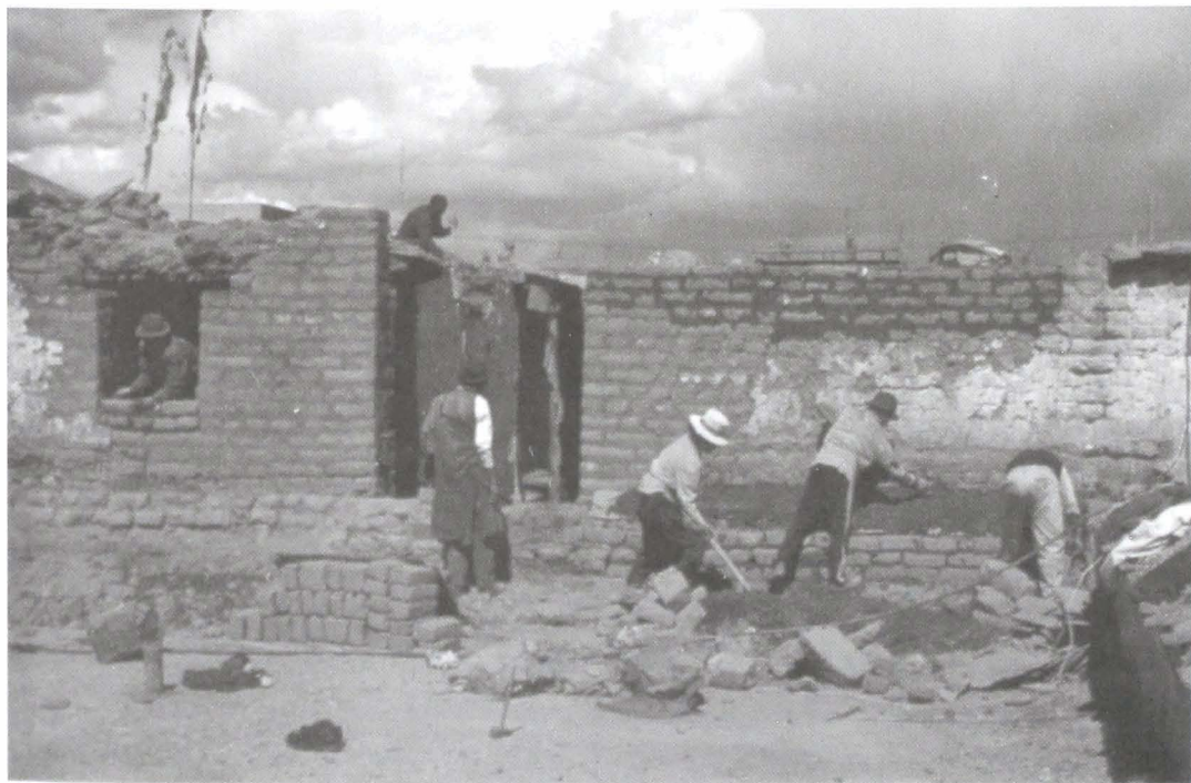
THF restoration works in Oedepug area
