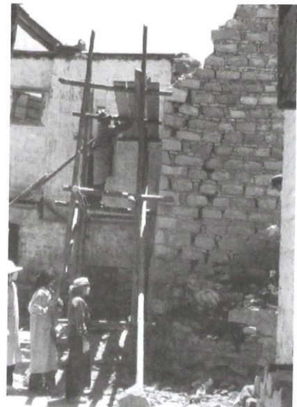
THF repair of Labrang Nyingba northern toilet
