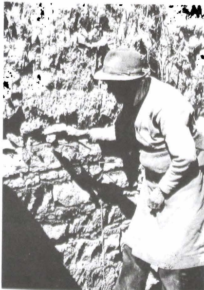
Building master Migmar, repairing southern wall of Nagtsagjang
