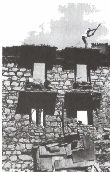
Demolition of northern wing of Tromsikhang, 1997
