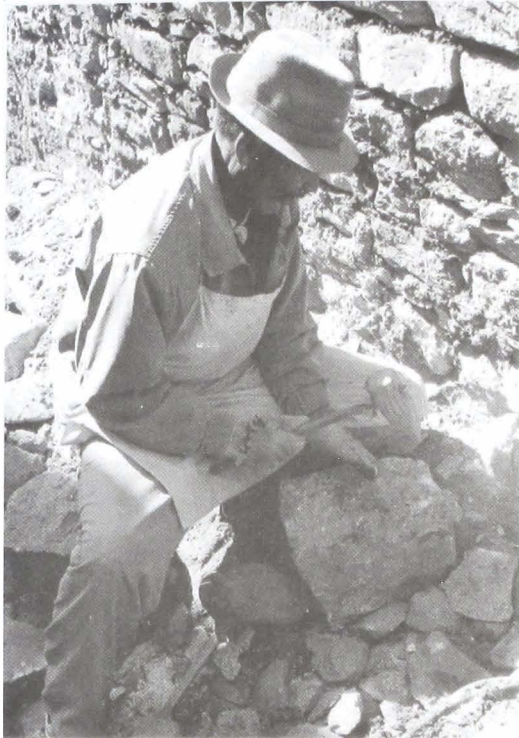
THF mason Loya cutting stones for repair of Nagtsagjang wall
