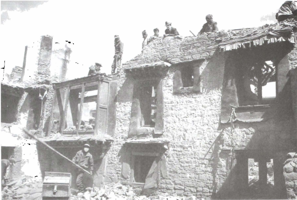
Demolition of 18th century Palling Liushar House, 1998
