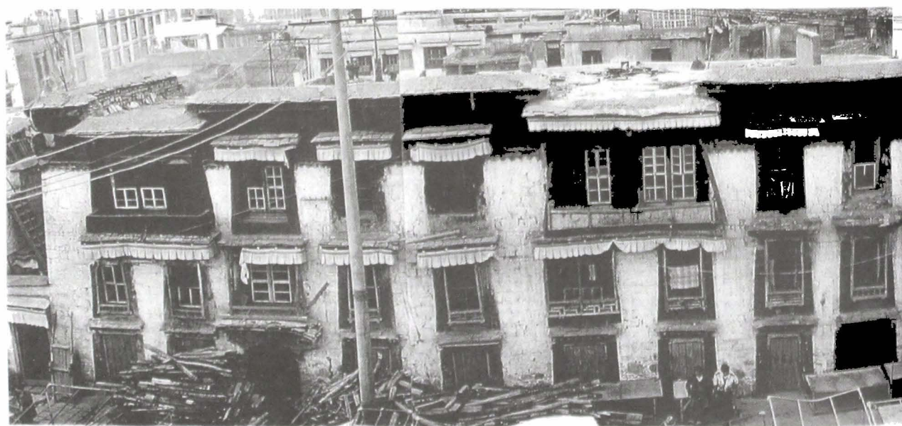
Tromsikhang, facade along Barkor Street, facing south, 1997
