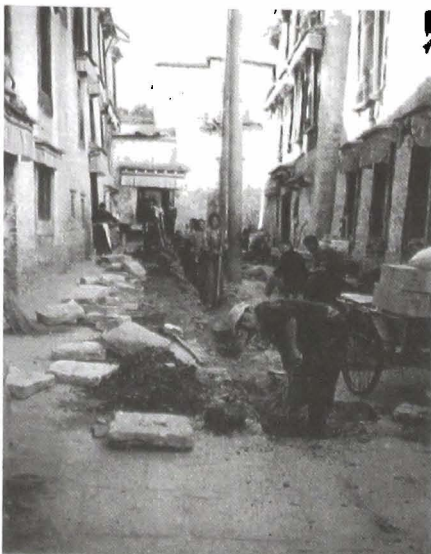
Workers digging trenches for THF water installations in conservation area
