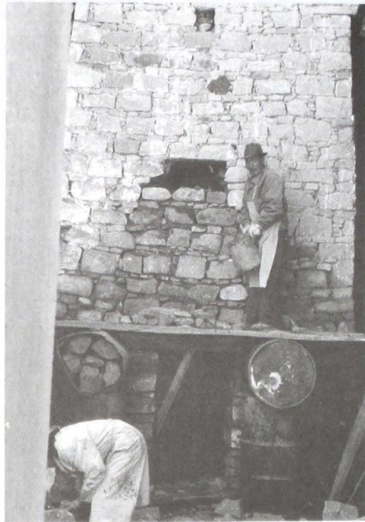
THF repair of Rongda toilet
