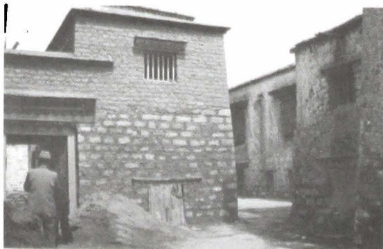
Juenpa house, THF toilet upgrading and restoration of main gate
